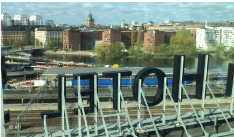
The hotel sign on the ninth floor of the Clarion Hotel Sign was firmly secured by a rack of hot dip galvanized steel.
