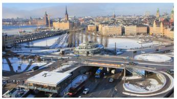
Winter picture of Slussen. Summertime there are a lot of greenery in the area that hide the overview. Slussen has an extensive bridge area, about 40,000 m<sup>2</sup>. This is divided into 24 bridge constructions.
