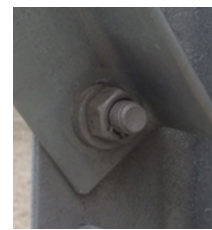
On the nut side, where a washer is used, there are no cracks.
