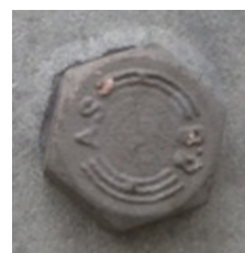
A small defect like this need no action.
