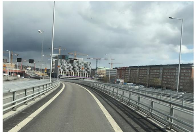
Bridge rails and fences in hot-dip galvanized steel on Norra Länken, recently opened for traffic in Stockholm.
