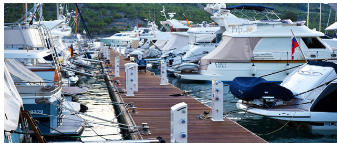
All-Concrete Pontoons are of exceptionally strong construction with a 50 year design lifetime. Aci Cres Marina, Croatia (Photo: Marintek)
