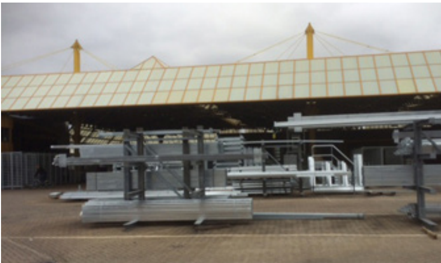
Verzinkerij Meerveldhoven has a large roof over the inner yard of the plant which means that no steel has to be stored outside when it is bad weather.
