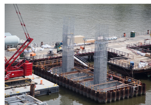
Over 27,000 tonnes of galvanized steel reinforcement ensures the long-term durability of the main span towers, approach span piers, abutments and road deck panels of the Mario M. Cuomo Bridge.
