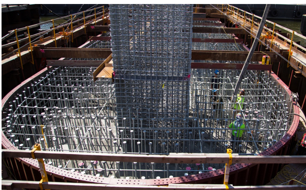
The 43 pairs of concrete piers of the Mario M. Cuomo Bridge are reinforced by galvanized reinforcing steel cages.
