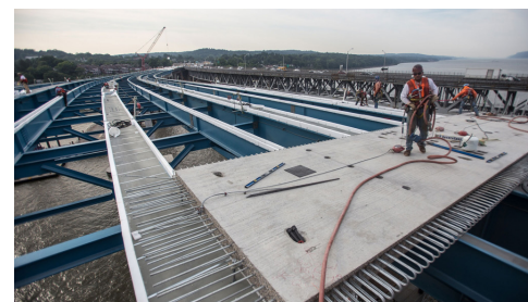
The bridge deck of the Mario M. Cuomo Bridge comprises nearly 6000 precast panels, each 3.66m long and 6.7-13.7m wide, for the approach spans and 963 main span deck panels. The panels are joined by pouring concrete around the protruding galvanized steel reinforcement. (Image courtesy of New York State Thruway Authority)
