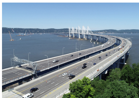
The Mario M. Cuomo Bridge is a 5km long, 8 lane twin-span cable stayed bridge designed for a minimum 100-year life using galvanized reinforcement.
