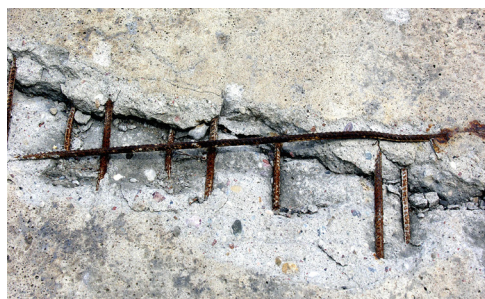
Cracking and spalling of concrete due to corrosion of the reinforcing steel
