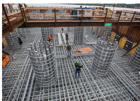
Prior to selecting galvanized reinforcing steel for the Mario M. Cuomo Bridge, the New York Thruway Authority developed a Corrosion Protection Plan to identify exposure, degradation mechanisms, design and construction strategies, and life-cycle costs.
